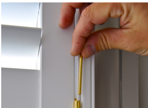
2 parts of hinge coming together with drop pin going in
